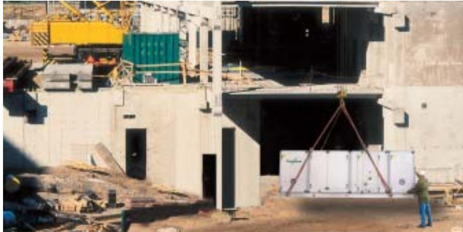
With placement outdoors the unit is fitted with a protective roof structure.
